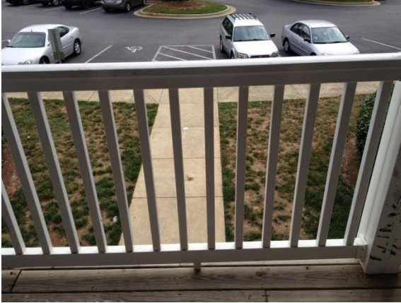
PVC railing in breezeways and stairways
