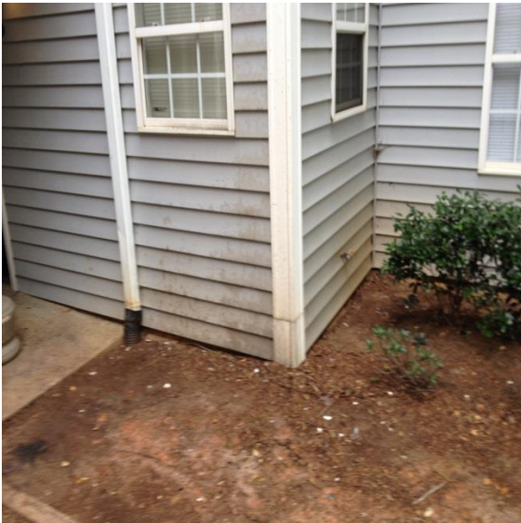
Photos showing condition of vinyl siding where gutters overflow onto the soil surface
