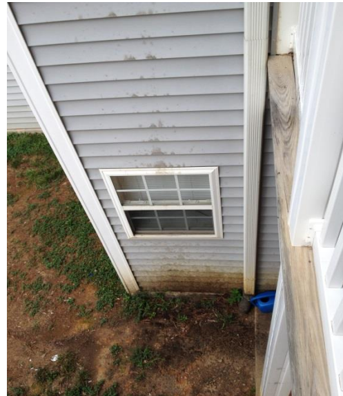
Photos showing condition of vinyl siding where gutters overflow onto the soil surface
