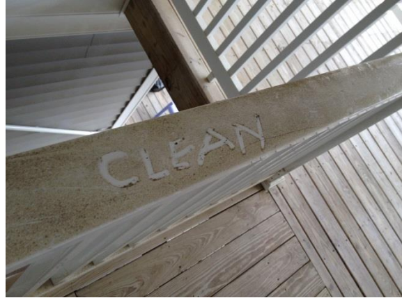
PVC railing in breezeways and stairways
