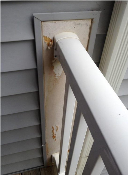
Rail connections showing deterioration with masonite (left) and vinyl handrail detached from wall (right)
